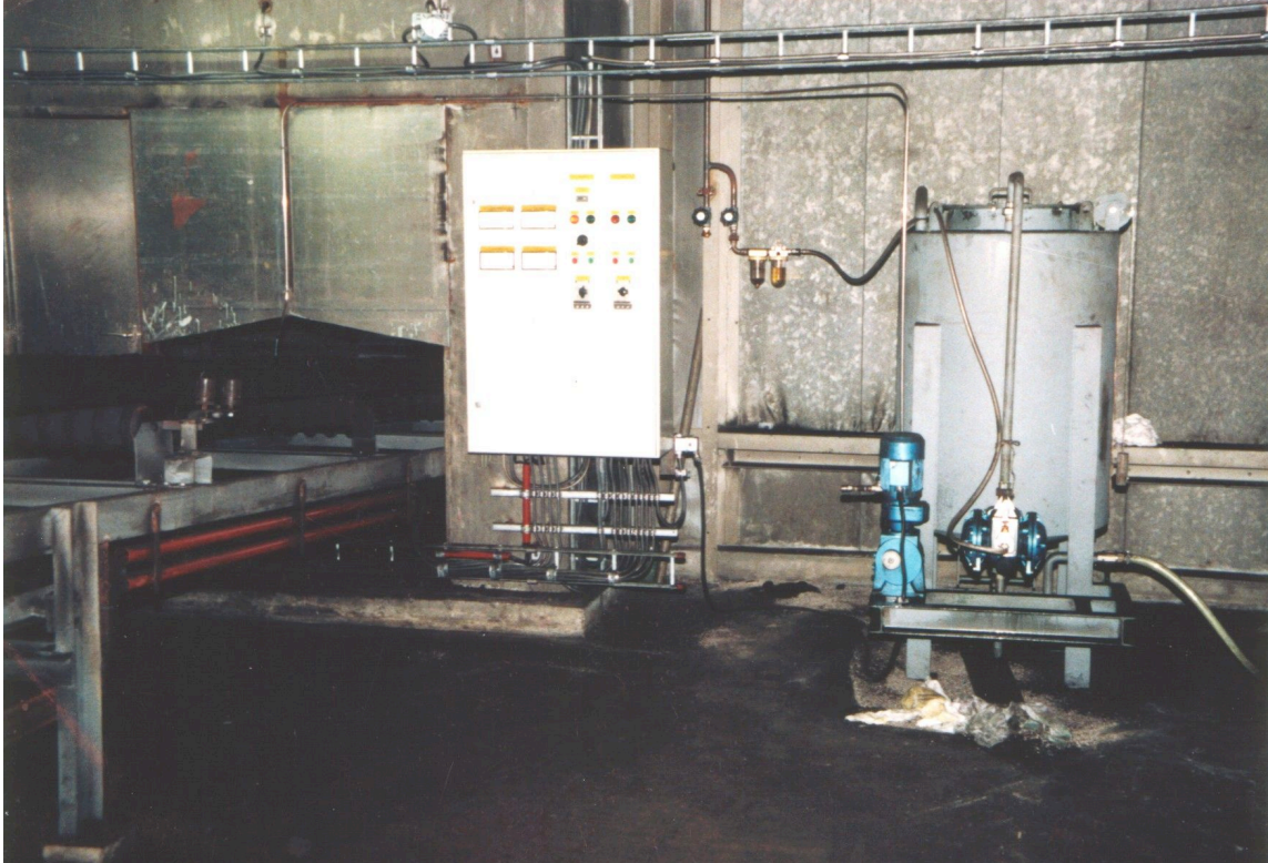
A small storage tank with dosing and recirculation pump is installed near the coal conveyor.
